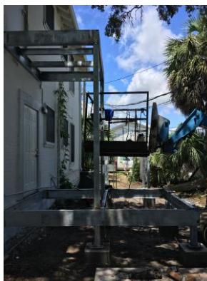
New stairway being installed behind the Carrabelle History Museum
